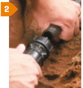
2 Ensure 2 threads are showing and simply slide the pipe in until the first point of resistance is felt.
