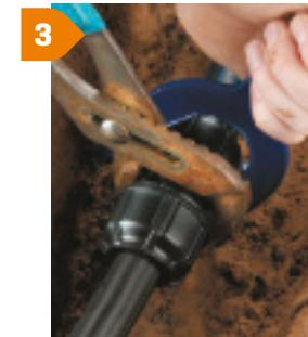
3 Tighten the nut by hand to the point where the nut is touching the flange on the body of the fitting. Do not tighten beyond this point.
