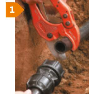
1 Cut the pipe square, there is no need to chamfer or lubricate
