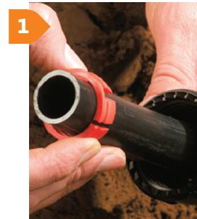
Cut the pipe square and place the nut and grip ring on to the pipe
