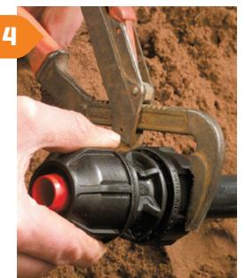
Tighten the nut with a wrench
