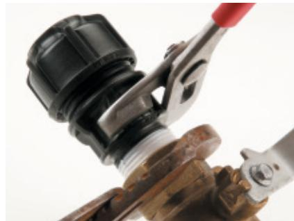
1. Apply PTFE tape or suitable\* sealant to the plastic thread ensuring sufficient is applied to ensure a watertight seal.
